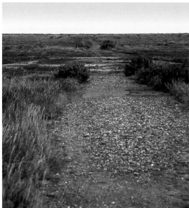
Fig. 4. A drove road at Warham Marsh. The example shown here has been surfaced with gravel, possibly during the Second World War.
