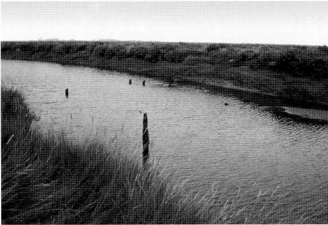
Fig. 5. The site of a former bridge at Warham Marsh. Wooden stumps are all that remain of the former supports for the bridge over a deeply incised creek.
