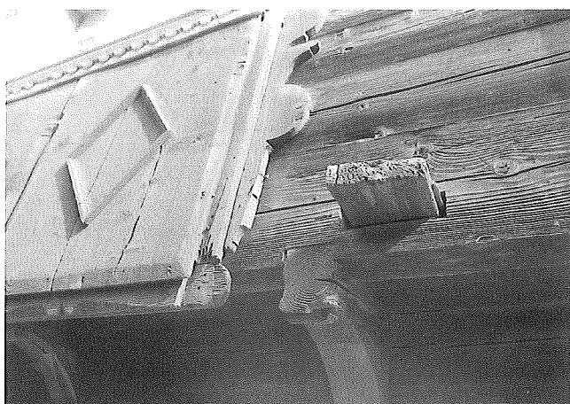
**Fig. 2.** Wedge plank for clamping internal floor planks tight. Silenen (UR), 17<sup>th</sup>/18<sup>th</sup> century. Photo B. Furrer 1980.
