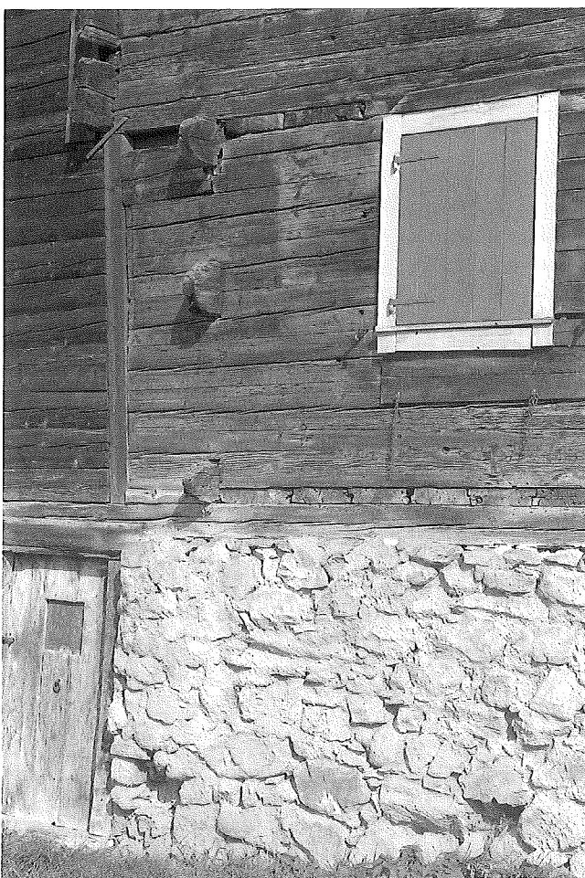
**Fig. 5.** Floor planks visible in elevation as well as irregular tie planks in a house in Morschach, Tannen, 1341d. Photo B. Furrer 1984.
