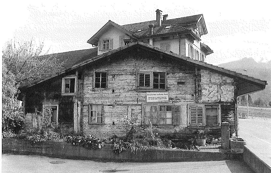
**Fig. 1.** Log building having floor plank ends visible on the exterior. No attic under ridgepole. House Nideröst in Schwyz, 117d. Photo B. Furrer 2000.
