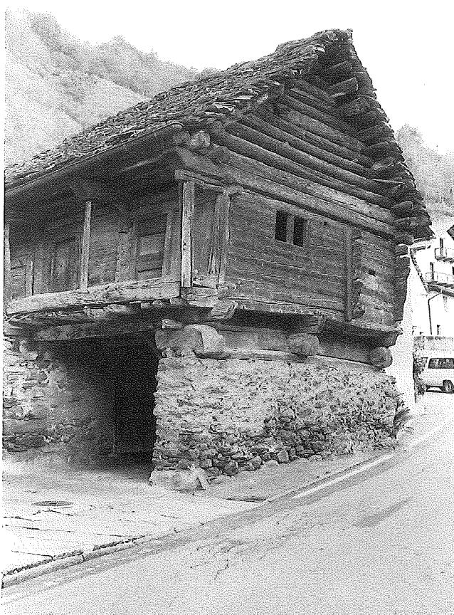
**Fig. 12.** Floor planks protruding on the side of a house to serve as gallery and access landing. Multipurpose farm house in Ponte Valentino (Blenio, TI). Photo B. Furrer 2001.
