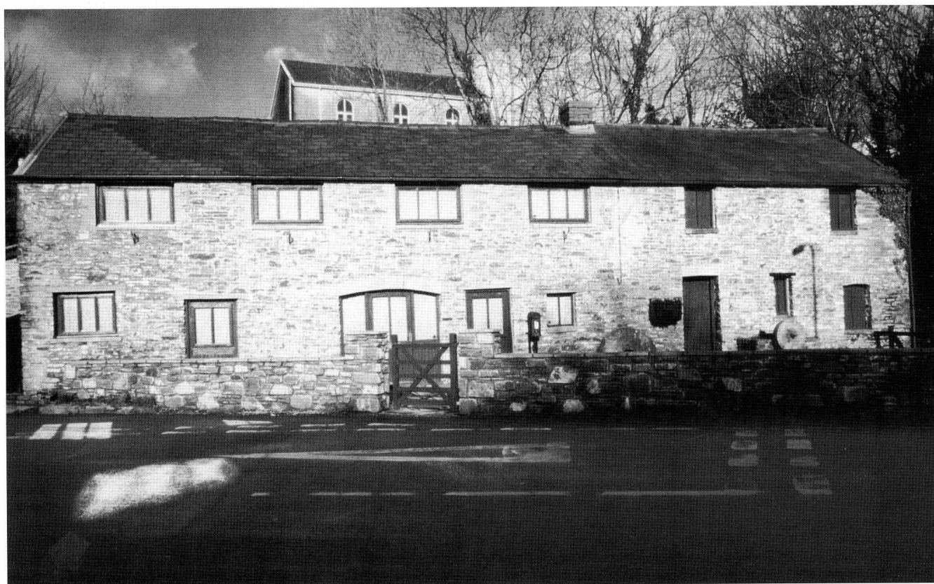
Fig. 3. The restored mill at Felindre. The leat runs behind the structure to turn a wheel which lies on the right hand side of the building as one is facing it.
