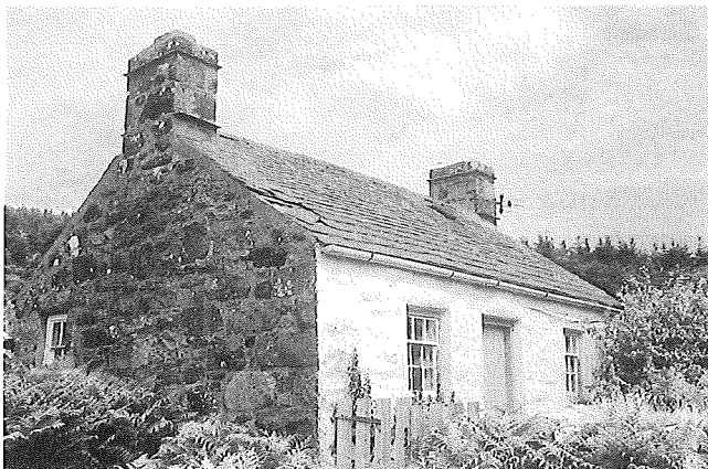
Fig. 4. Limewash and slate in a small cottage, Llyn, North-west Wales.
