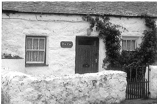
Fig. 6. Limewash and sash windows in a small roadside dwelling, Llyn, North-west Wales. (All photographs are Cadw: Welsh Historic Monuments).
