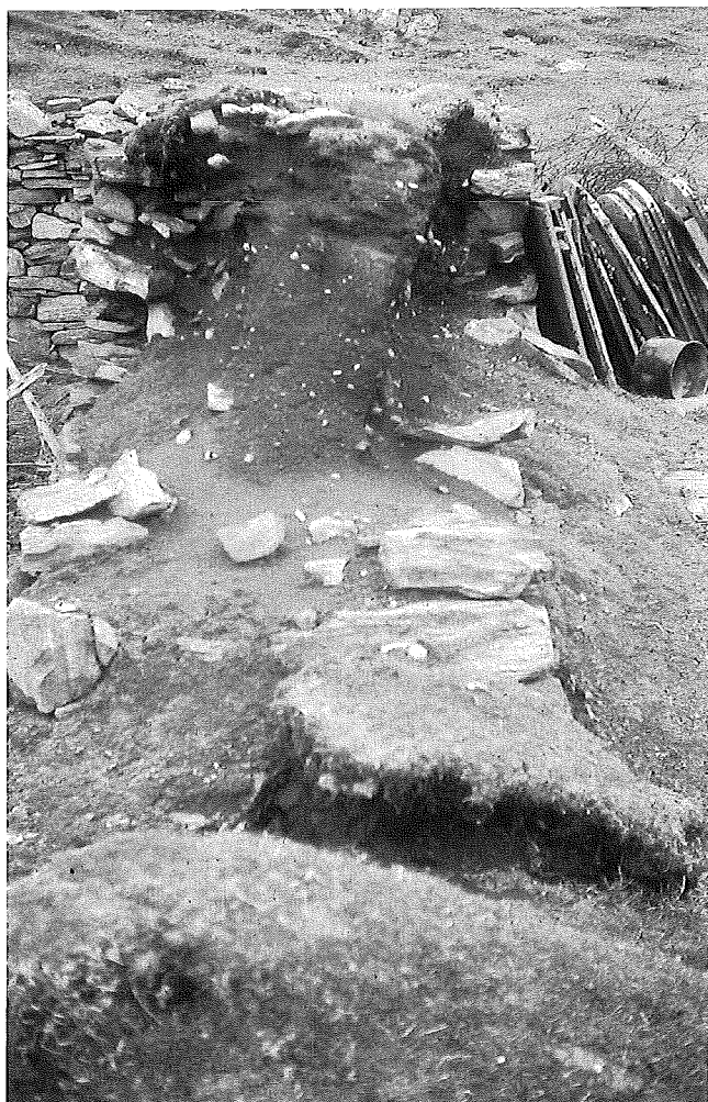
Fig. 4. The so-called 'double-walled' construction in section from a blackhouse at Carloway, Lewis, showing the earth core. Crown Copyright RCAHMS.
