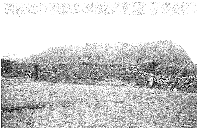
Fig. 5. View of a blackhouse at Carloway, Lewis showing the hipped roof resting on the inside of the walls. Crown Copyright RCAHMS.
