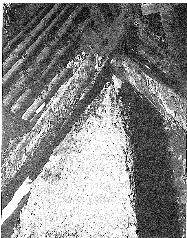
Fig. 7. A closed single-blade cruck at Achcullin, Inverness-shire showing the crossed apex for the ridge-tree. Crown Copyright RCAHMS.
