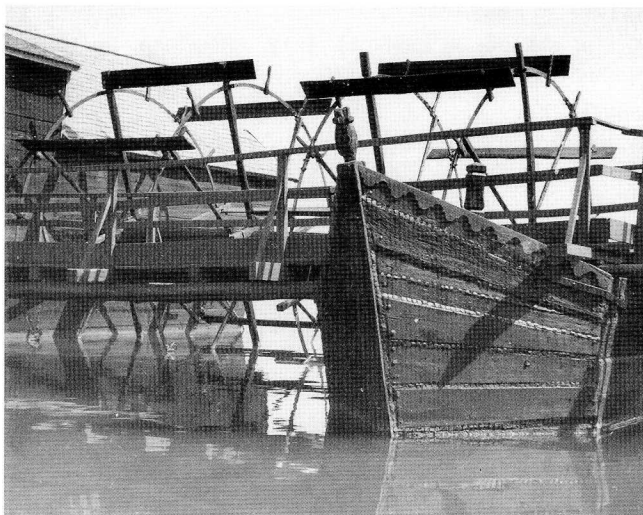
Fig. 13. The water wheel of a ship mill (Ráckeve, river Danube).
