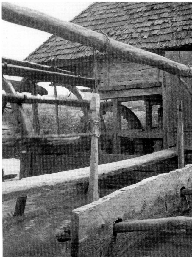
Fig. 10. Wooden lock to stop the water wheel (Sülelmed – Kelence 1942).
