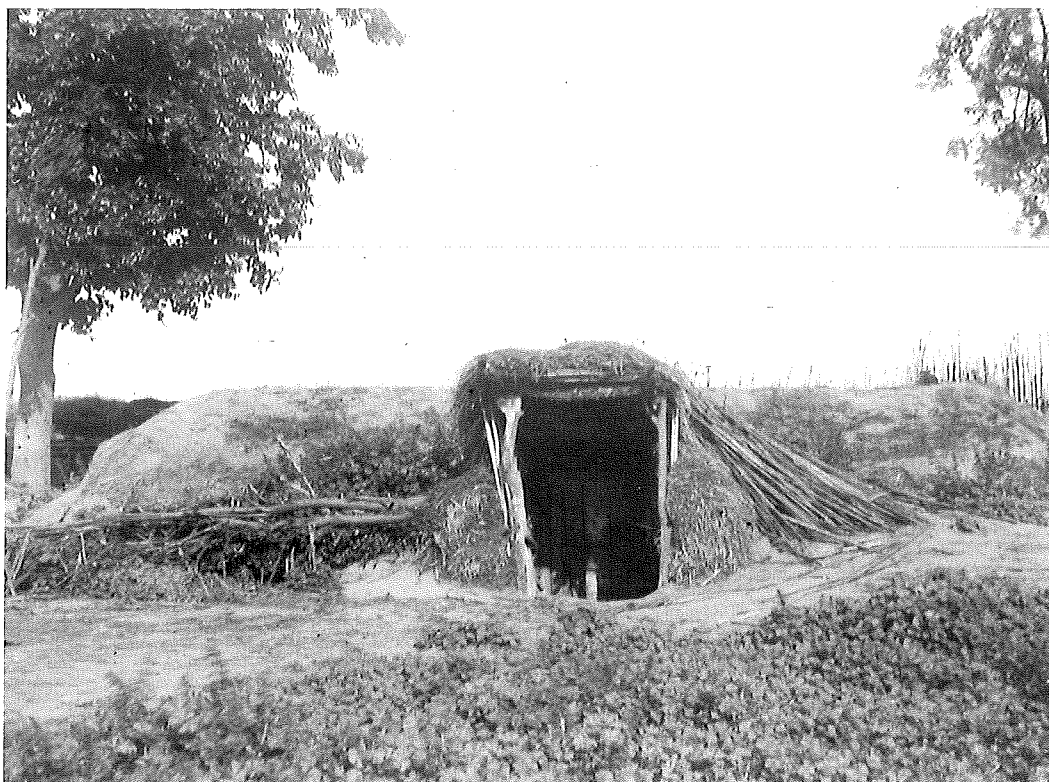
Fig. 15. Semi-subterranean stable with small roofed entryway in Balkány (Photo by Tagán Galimdsán, 1933).
