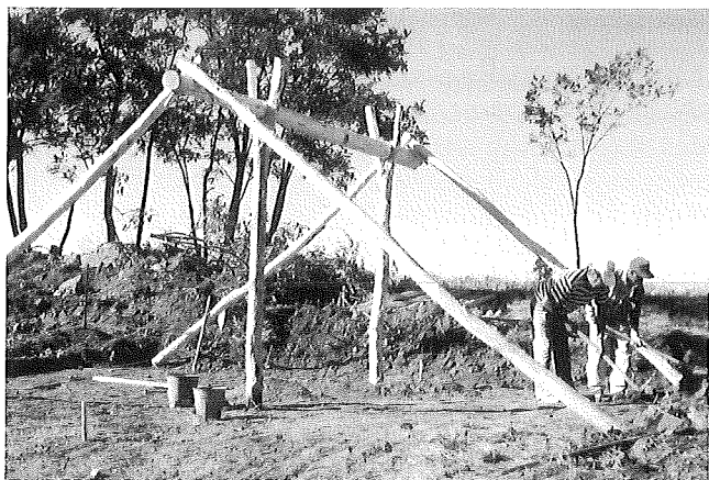
Fig. 16. Setting up the structure of the pit house (Photo by T. Sabján 1997).
