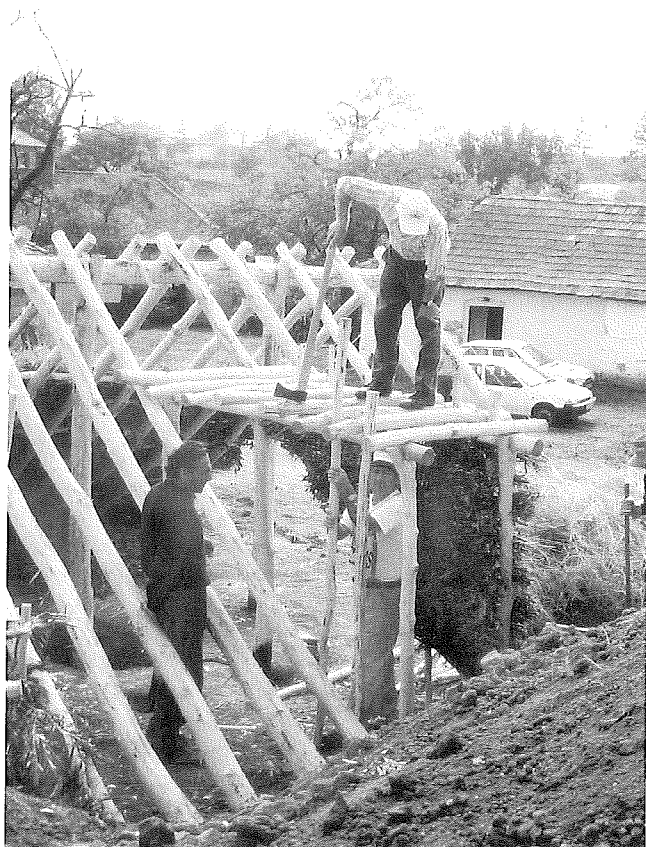
Fig. 17. Covering the roof with earth.
