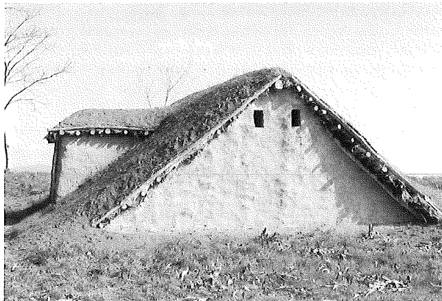
Fig. 18. The pit house under its finished roof.
